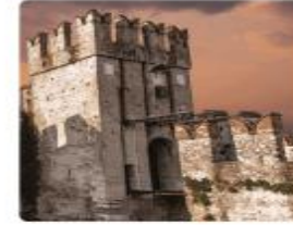
Towers, Tunnels and Turrets
